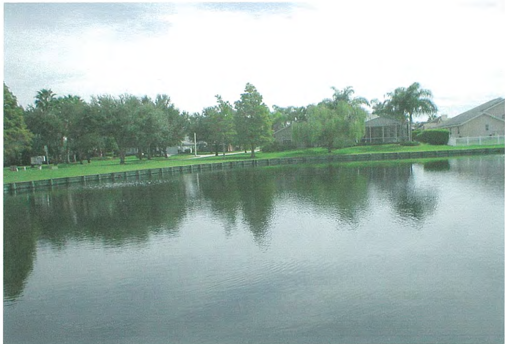
EXISTING RETAINING WALL
